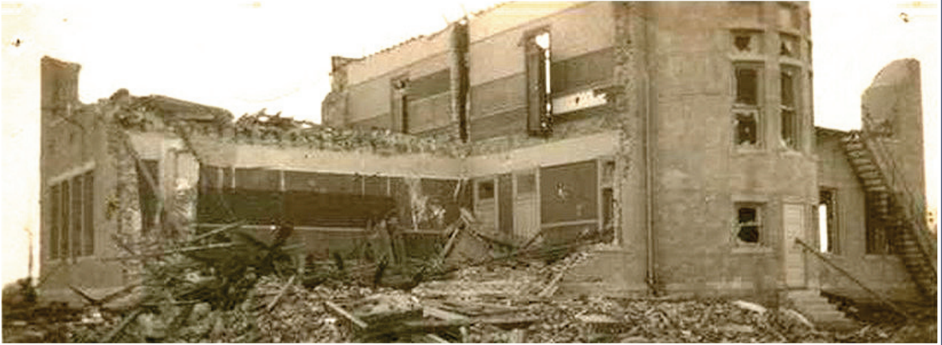
East Side of Roosevelt school damaged beyond repair by the Nov. 10, 1915 tornado.
