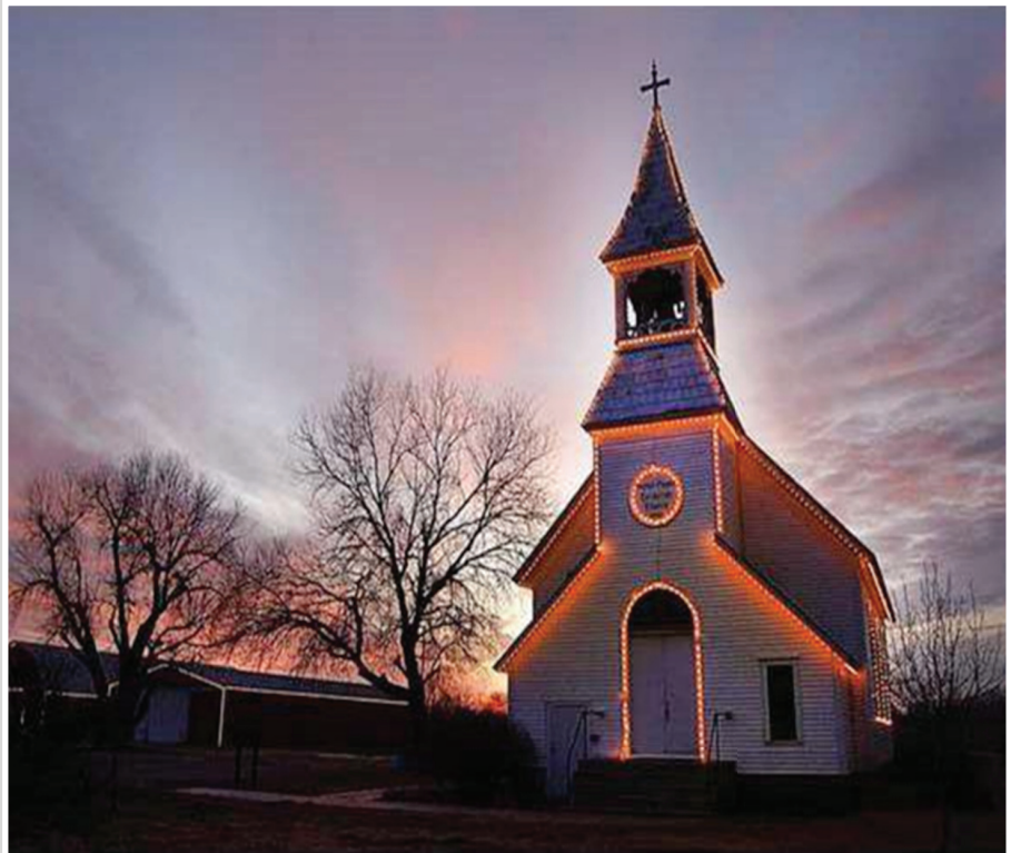
First was the former St. Paul's Lutheran Church, which was moved to the site in 1967.
